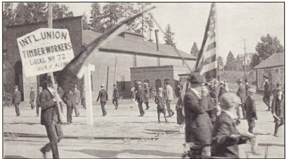
International Timber Workers, Local 72 near 1st & Sherman, 1919. Lab-5-29
